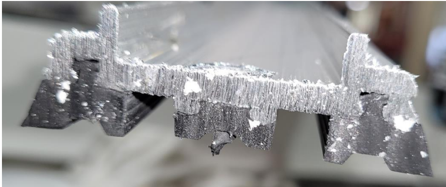
Photo No. 6 Pressure plate profile
