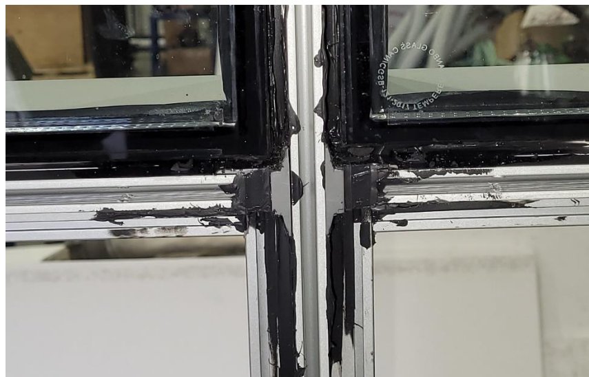
Photo No. 14 Mullion joint
