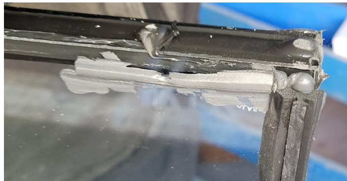
Photo No. 10 Interior glazing gasket with silicone at corners
