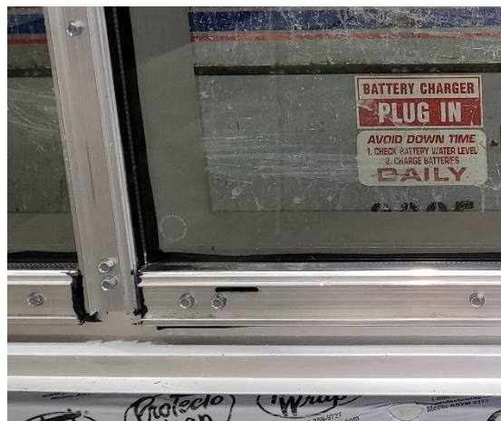
Photo No. 11 Pressure plate fasteners and drain slot
