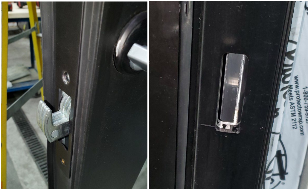
Photo No. 11 & 12 Hook Lock, left; Keeper Slot, right
