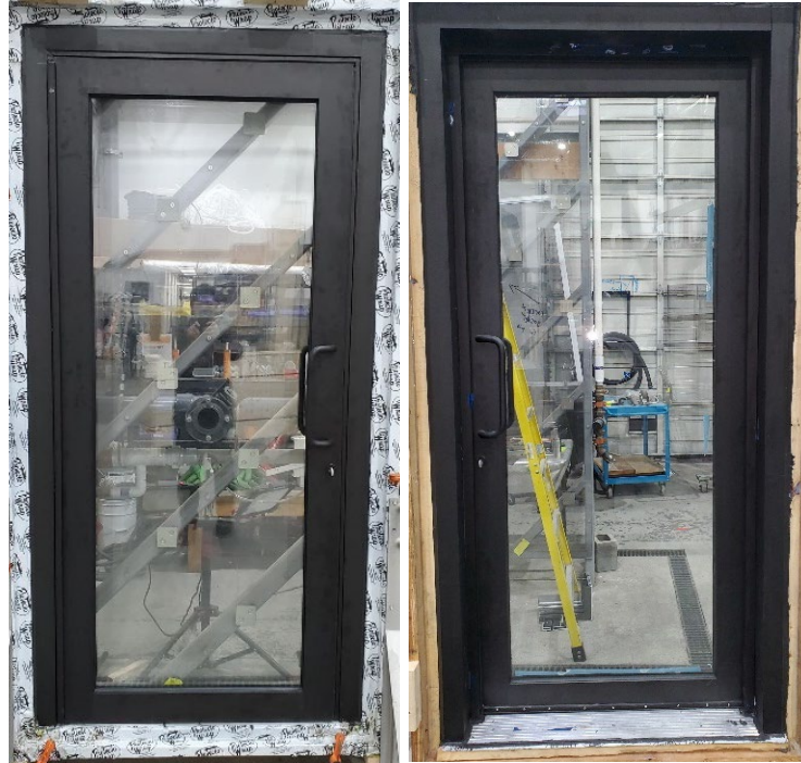
Photo No. 1 & 2 Outswing Side-hinged Entrance Door – Exterior, left; Interior, right
