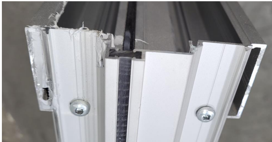
Photo No. 7 Corner joint fasteners for one side of vertical mullion
