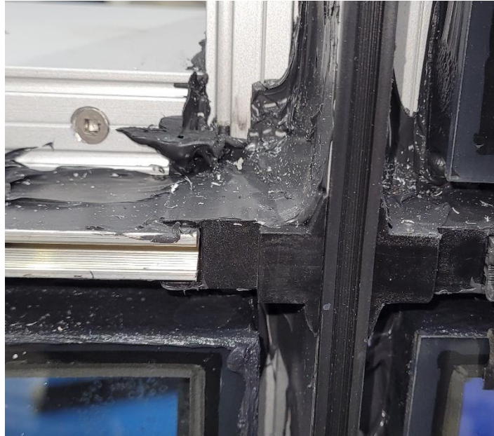
Photo No. 15 Mullion joint with spacer blocks
