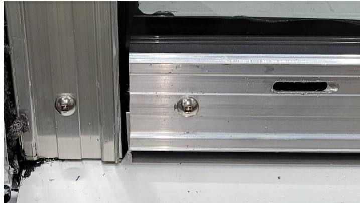
Photo No. 10 Pressure plate joint, bolts and drain slot
