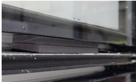
Photo No. 17 Setting blocks
