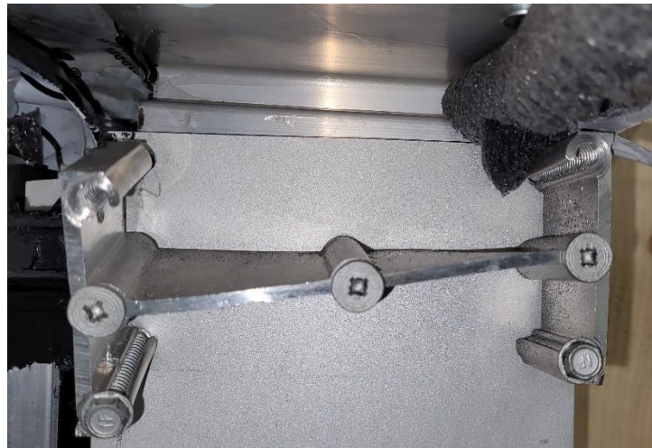
Photo No. 12 Aluminum shear block secured to the jamb
