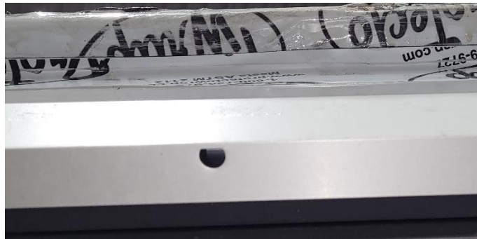
Photo No. 16 Beauty cap drain hole
