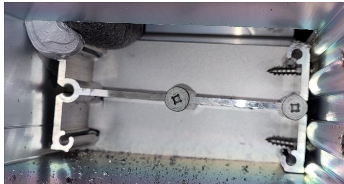
Photo No. 11 Aluminum shear block secured to the mullion
